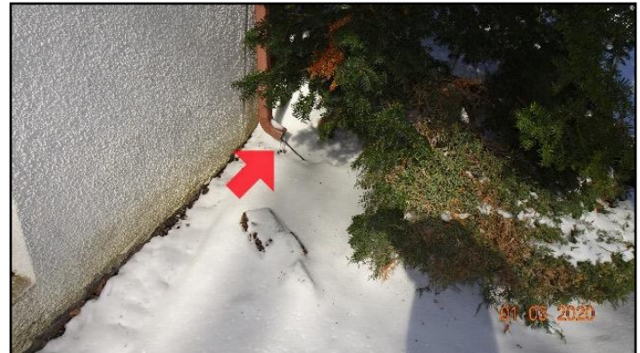
4. Should discharge 6 feet from building
