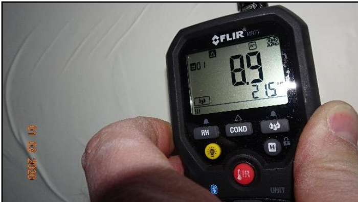
44. Moisture meter reading
