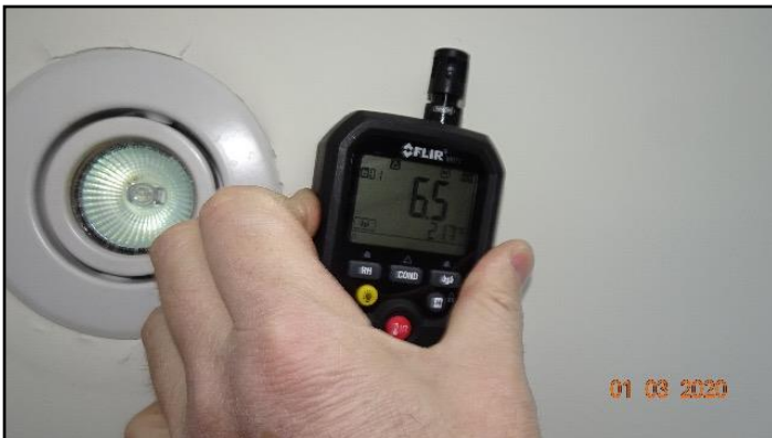
42. Moisture meter reading
