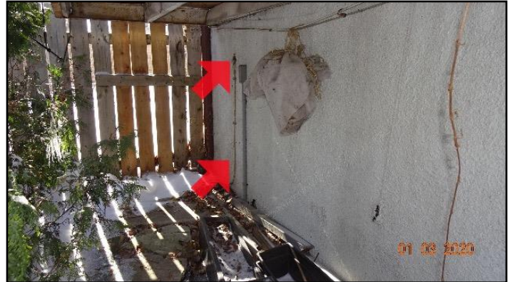
18. Wire not protected
