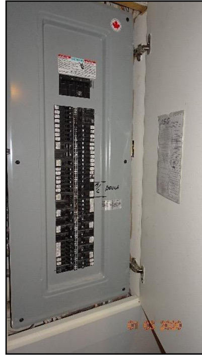
16. 200 Amps Distribution panel
