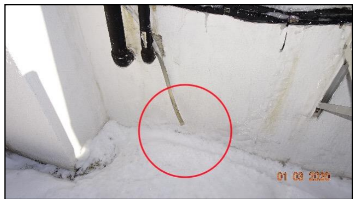
33. Improper discharge point
