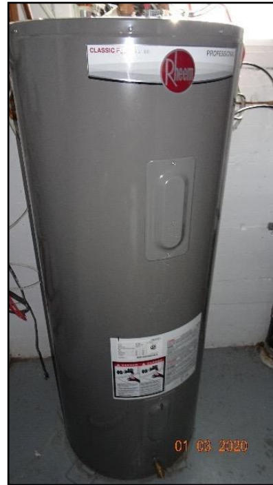
38. Water heater I
