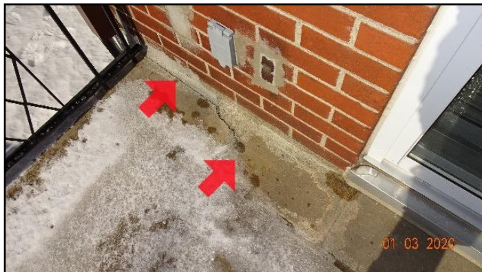
11. Cracked floor
