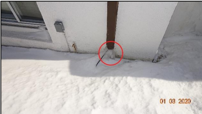
3. Should discharge 6 feet from building
