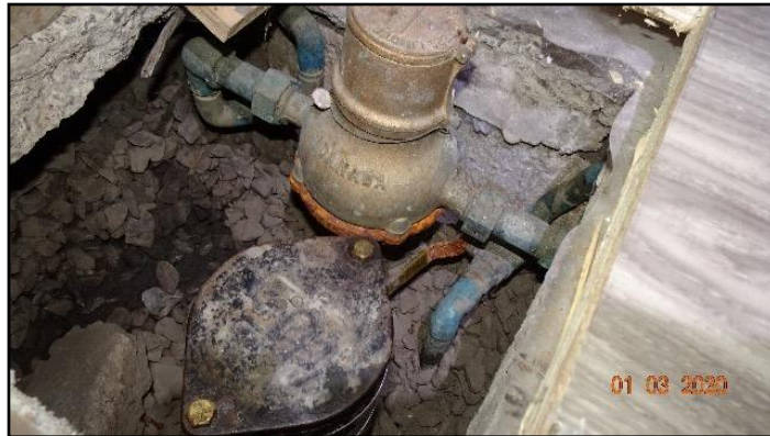
39. No seal on water meter
