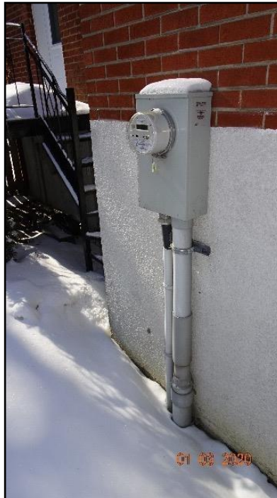
13. Underground Service entrance
