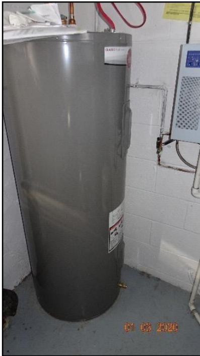
37. Water heater II
