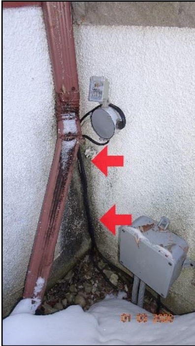
17. Wire not protected
