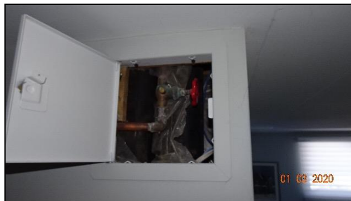
36. Main water shut off valve
