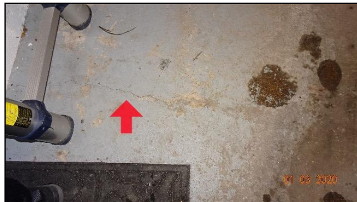
49. Cracked floor
