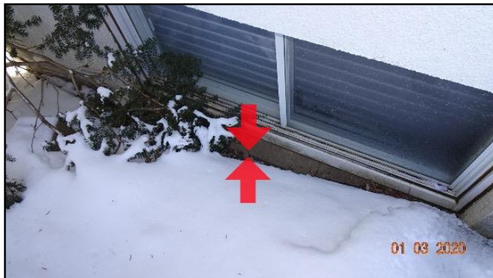
10. Missing window well
