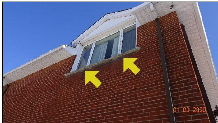
9. Sill deteriorated
