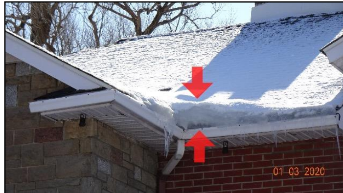
1. Vulnerable to ice damming
